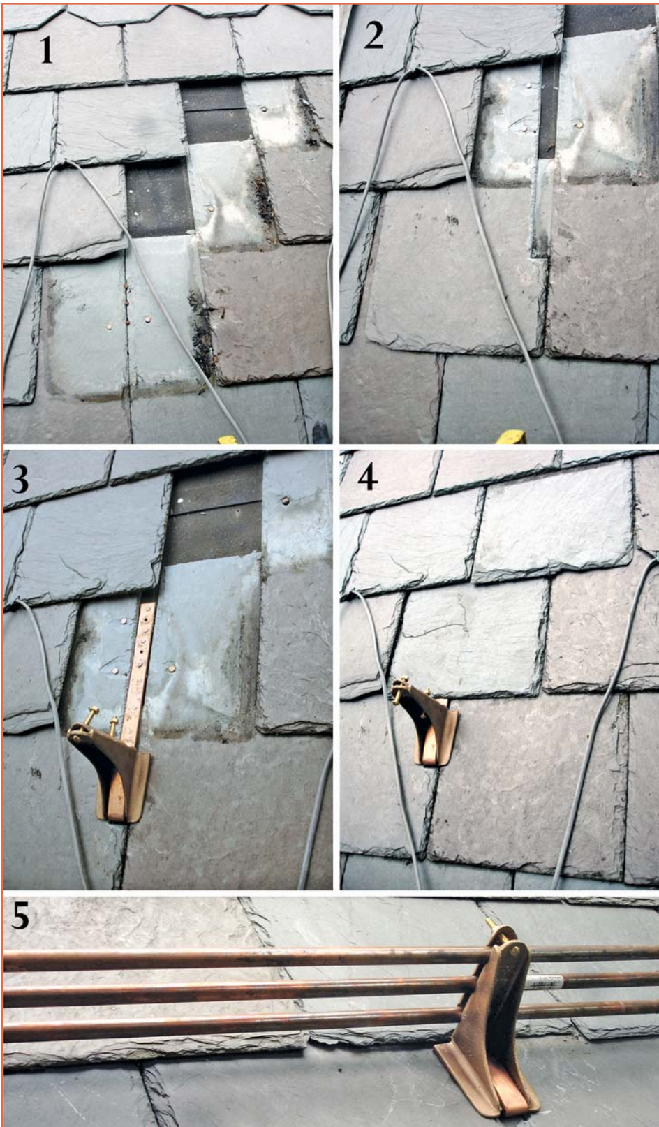
Figure 11 – Snow guards with shafts can be added to existing slate roofs if some of the slates are removed, as illustrated in this series of photos: 1) Remove three diagonal slates, the lowest of which will be the slate underneath and to the left of the snow guard. 2) Notch the lowest slate and reinstall it using two nails on the right side, one above the other. 3) Insert the snow guard shaft into the notch and fasten it to the roof deck using nails or screws. 4) Insert the slate immediately above the snow guard and fasten it with two nails on the right side. Then insert the third slate and fasten it with a slate hook. 5) In this case, the snow guard is a rail bracket. Such brackets only need to be installed in a single row and are spaced approximately every three slates.
