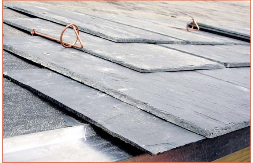
Figure 5 – Copper “loop-the-loop” snow guards are perhaps the least expensive of all snow retention systems. They’re easy to install and effective when used in sufficient quantities.
