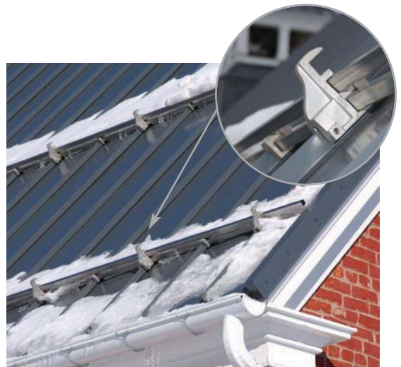
The roof on this church details the use of the Berger "F-Rail"™ Snow Retention System
