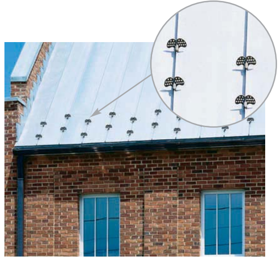
The roof on this church details the use of Berger cast aluminum "RT Snow Guards".
